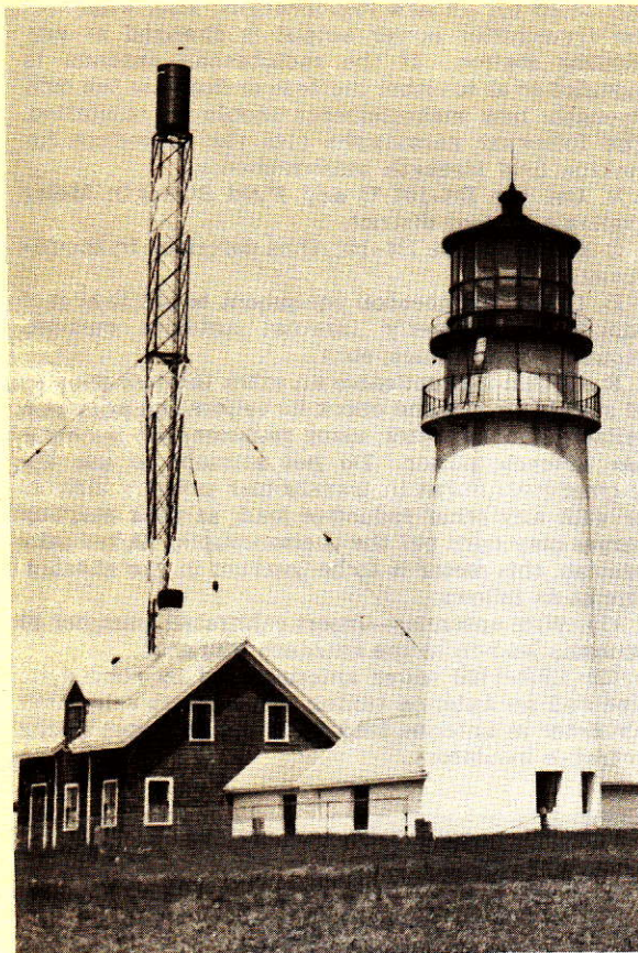
FIGURE 26-32.—LSR-1101 antenna at Cape Cod Light Station, Mass.
