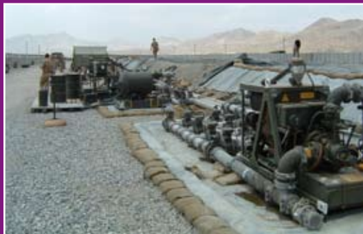
Fuel Pump and Filter Installation
