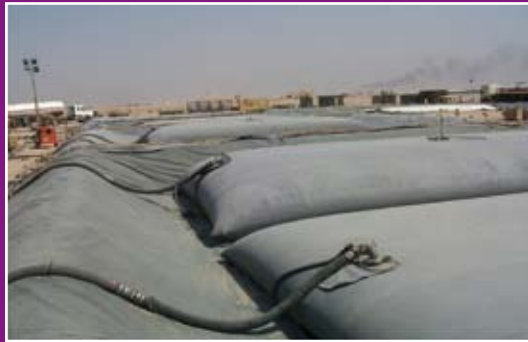
Deployable Fuel Handling Equipment for Expeditionary Operations Main Bulk Fuel Installation at Kabul International Airport, International Security Assistance Force (ISAF)
