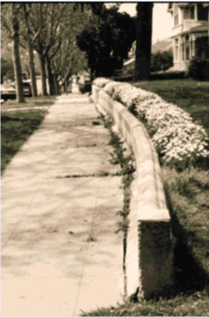
Left: Creeping along the Calaveras fault has bent the retaining wall and offset the sidewalk along 5th Street in Hollister, California (about 75 km south-southeast of San Jose). Right: Close-up of the offset of the curb. (Photographs by W. Jacquelyne Kiouss.)
