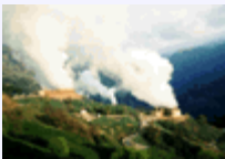
Geothermal powerplant, The Geysers [60 k]
