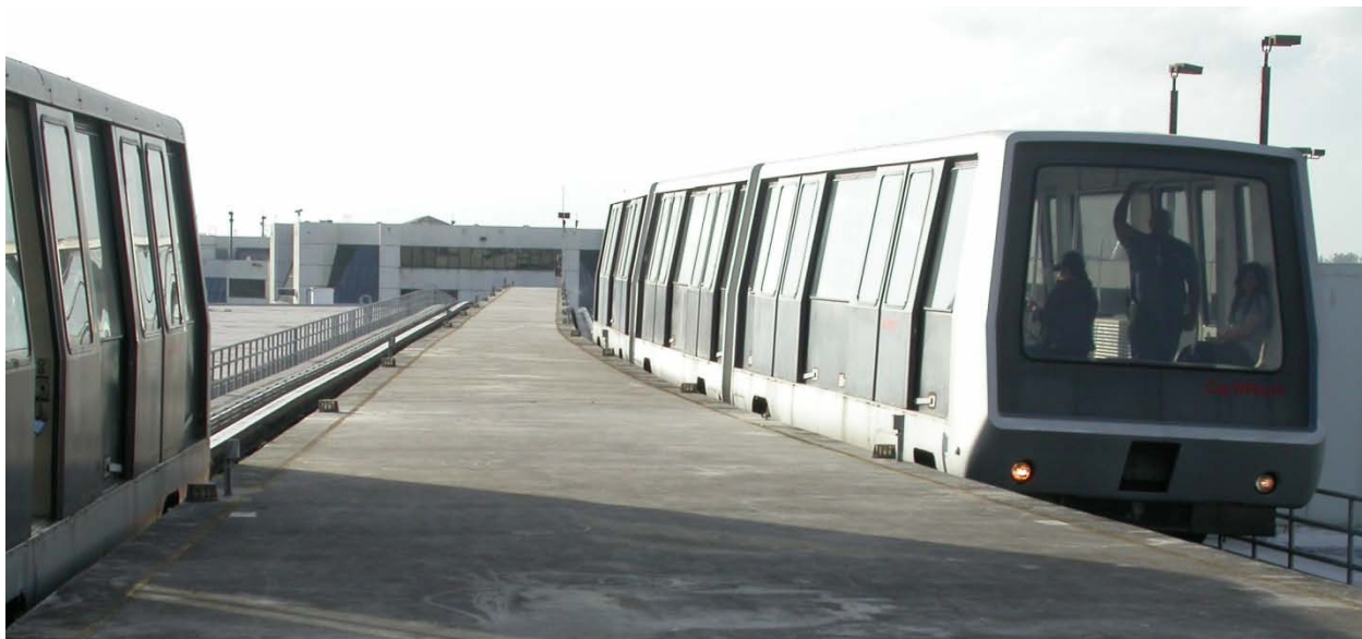
Figure 2. APM trains of the type involved in this accident. In this view, looking west toward Satellite E, the south train is on the left.
