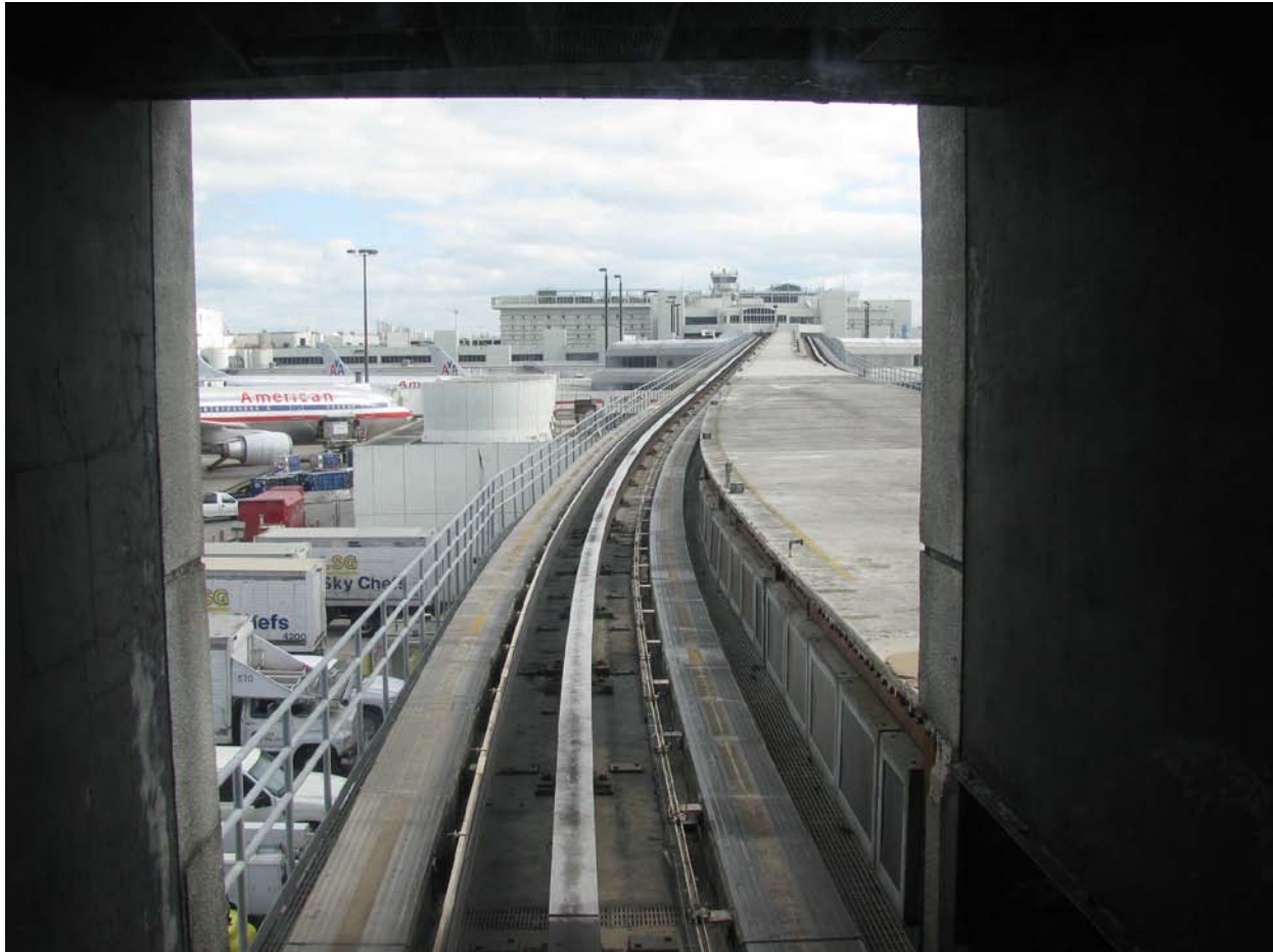
Figure 3. APM north train guideway looking toward the main terminal.
