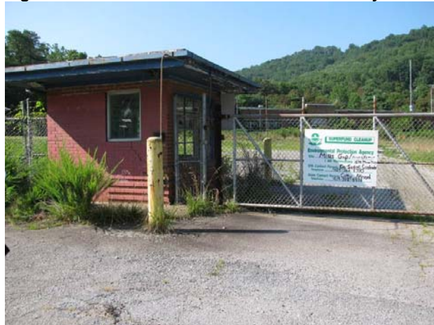
Figure 1: Entrance Gate to Former CTS Facility
