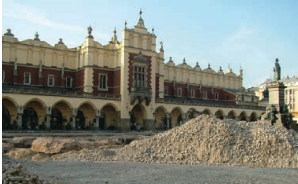
Slag Recycling, a Clean Business company, specializes in turning waste from what was Europe's largest steel plant in Krakow's Nowa Huta district into building material, used for example to repave Europe's largest medieval square, above, also in Krakow. The result is transport cost and environmental savings, thanks to turning local waste into resources for new construction.
