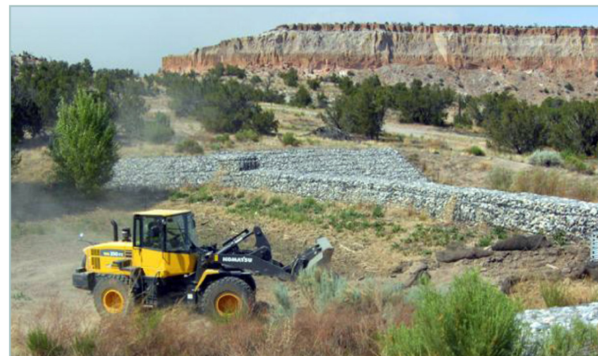
Figure 1-5. Heavy equipment working near a weir
