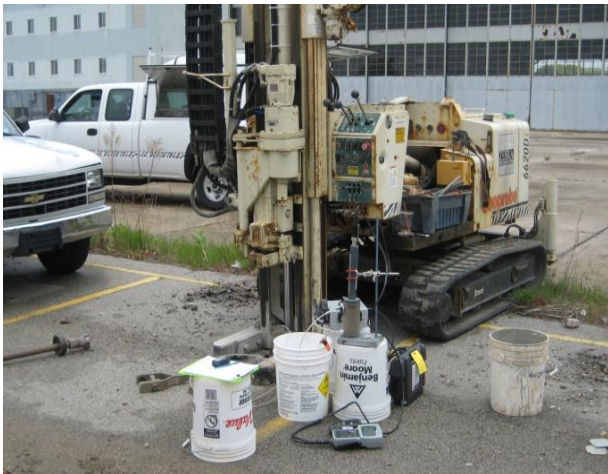
Figure 4 – Groundwater Profiling, Spring 2009
