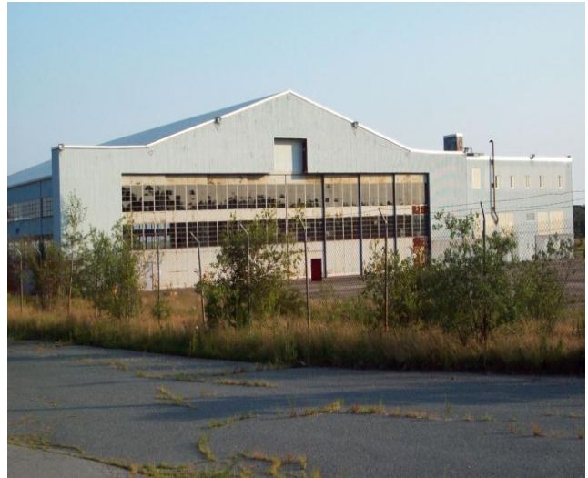
Figure 2 – Present View of Building 82 Facing South
