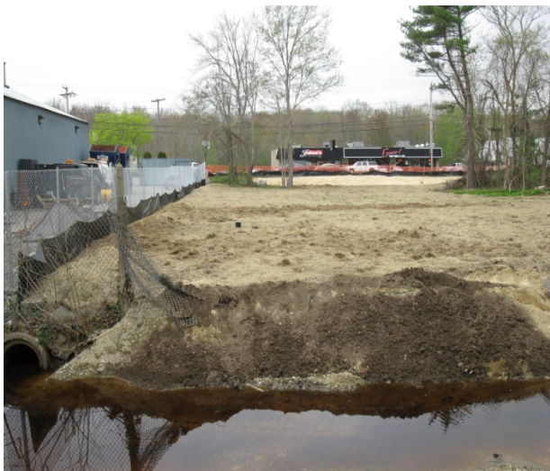
Figure 3 – Site After Removal Action, May 2011
