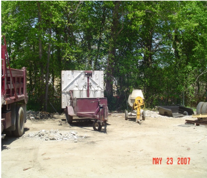
Figure 2 – Site During Initial Site Visit, May 2007
