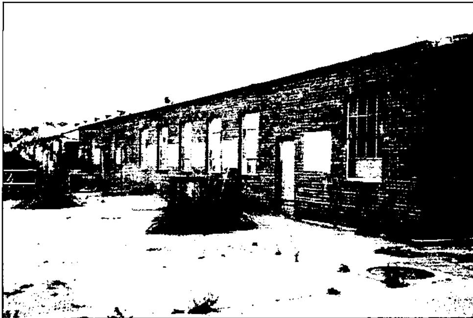
Tool and Paint Building (Building 207)
