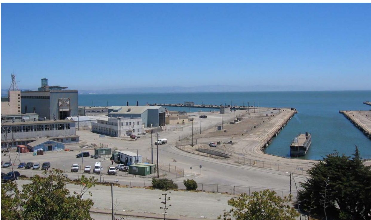
Viewpoint A: View Southeast from HPS Phase I Hilltop Park (Parcel A)
