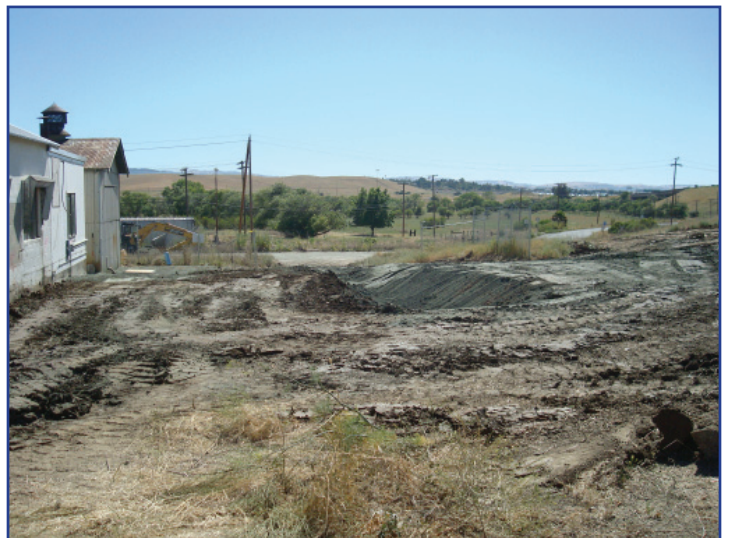
Site 27 restored to original grade after the TCRA
