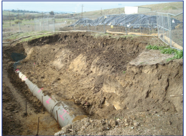
Site 27 TCRA excavation pit
