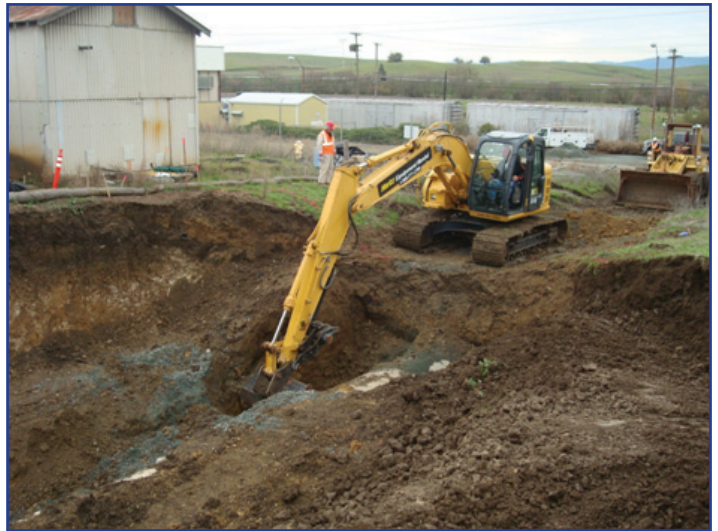
Removing contaminated soil at Site 27
