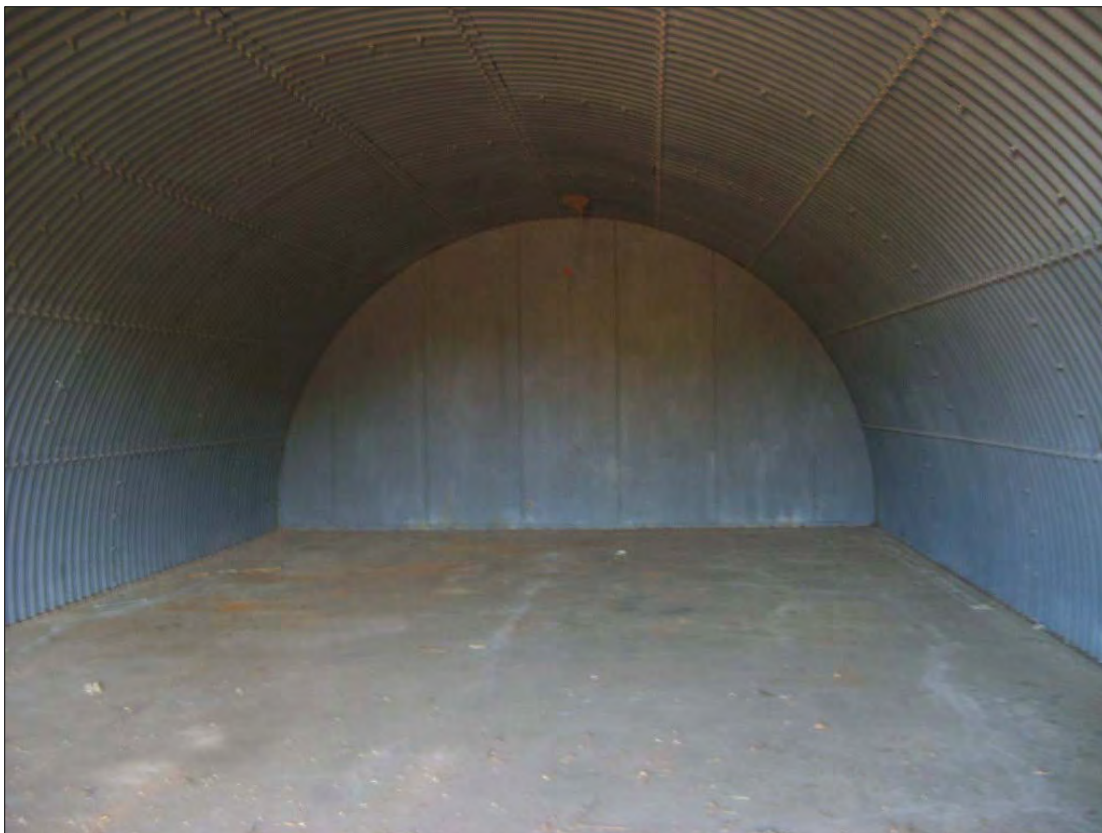
2. Building 1493 interior, view facing north.
