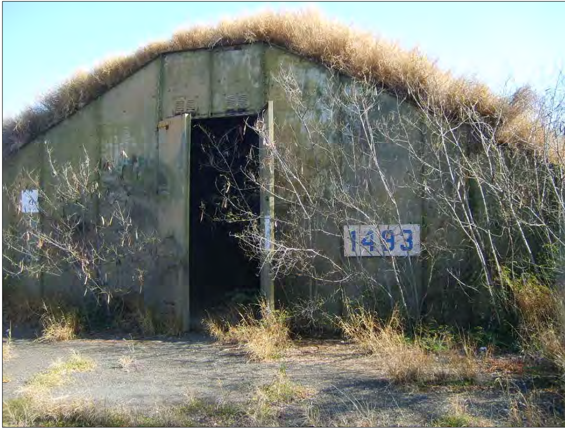
1. Building 1493 southern exterior concrete wall, view facing north.
