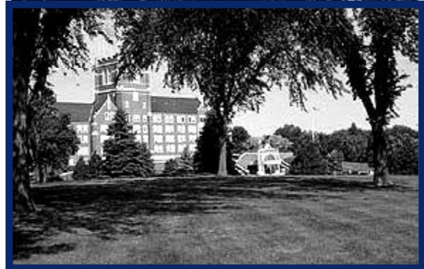
VA Medical/Regional Office Center Sioux Falls, SD
