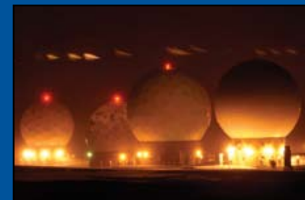
These "golf ball" protective covers at Thule Air Base, Greenland, house satellite dishes used to communicate with orbiting satellites.
