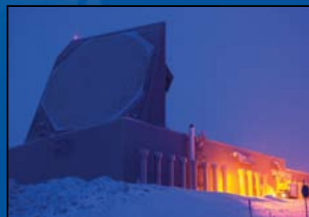
One of the two radar faces of the Ballistic Missile Early Warning System at Thule Air Base, Greenland.
