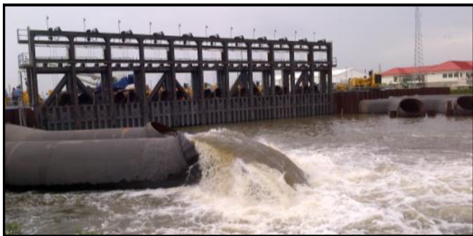
Operation of the 17th St. Canal Flood Gate pumps during Hurricane Isaac.
