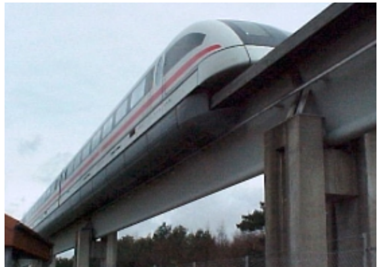
The TR-08 three-section Transrapid train at the test facility in the Emsland region of northwest Germany.
