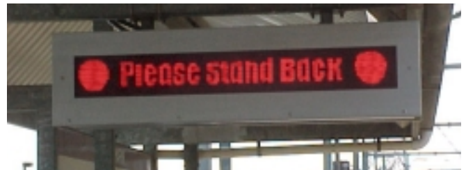
TAMS is a visual and audio warning system that alerts people on the platform when a train is approaching.
