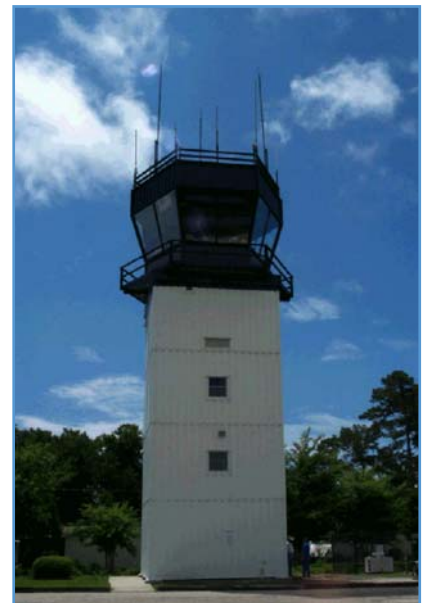
A Volpe team conducted evaluations of code compliance at four air traffic control towers including this tower in North Myrtle Beach, South Carolina. (Photo courtesy of Mr. Mark Gentile)
