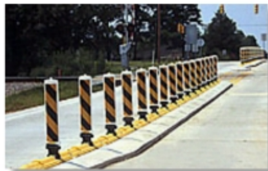
North Carolina DOT believes that median barriers have proven to be a low-cost investment with a high rate of return in safety at grade crossings. The barriers reduce drivers' ability to drive around lowered gates.
