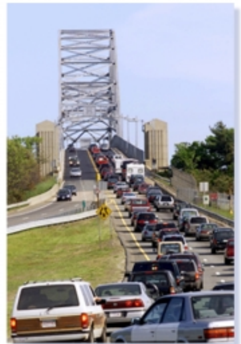
Most visitors to Cape Cod use one of two bridges that connect the Cape to Southeastern Massachusetts. Bottlenecked summertime traffic, as shown above, can detract from the relaxing atmosphere people seek. Recently, the Cape Cod Regional Transportation Authority voted unanimously to adopt all of the Volpe Center's early-implementation recommendations to improve public transportation to, from, and on the Cape starting this summer.
