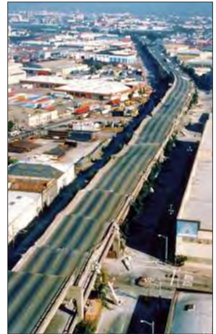
This collapsed California freeway is an example of the effects an earthquake can have on infrastructure.
