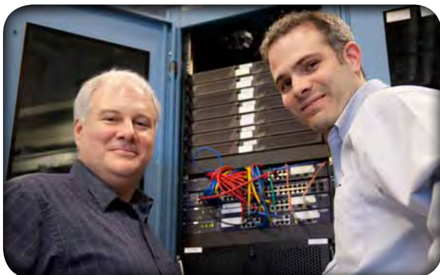
Steve Miller (left) and server administrator John Quigley in the storage area network server room.
