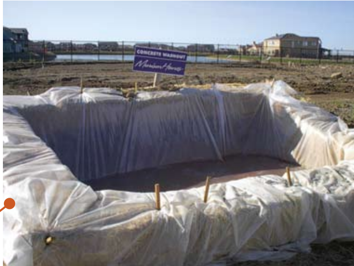
Photo 1: Well-maintained and labeled concrete truck washout
