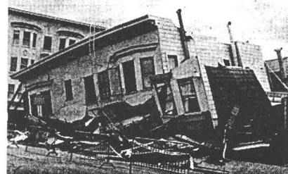
A crumbled house after the Loma Prieta quake in San Francisco in 1989.
