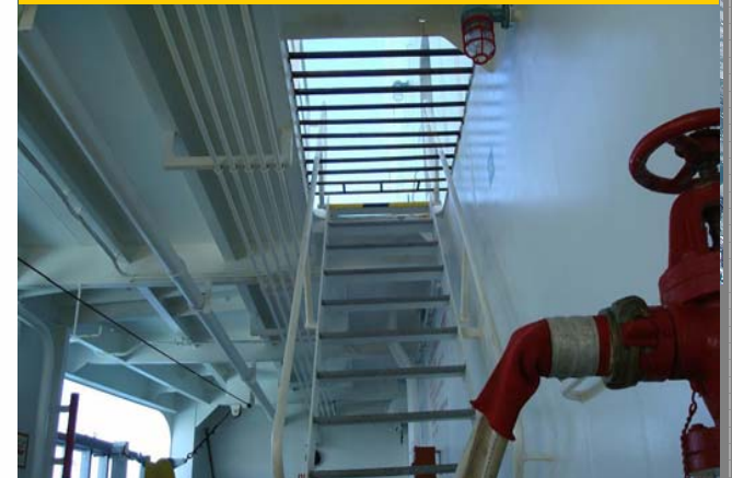
Onboard control areas secured
