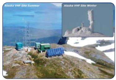
As shown by this remote Alaska tower site, construction season, accessibility for maintenance and repairs, equipment structure and durability are all challenges faced in Rescue 21 Alaska system design and deployment.
