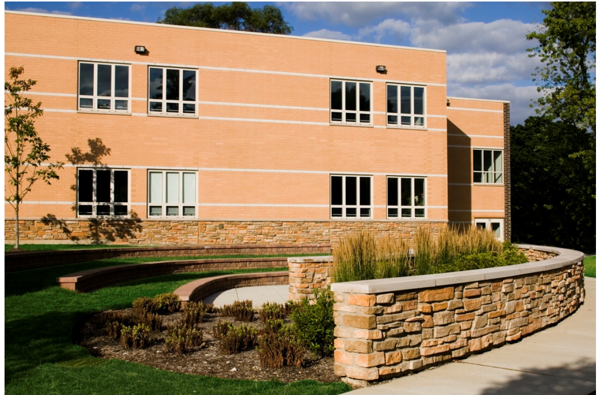
► Winfield School Addition, FGM Architects, Winfield, IL
