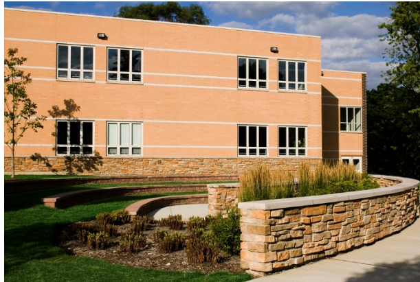
▶ Winfield School Addition, FGM Architects, Winfield, IL
