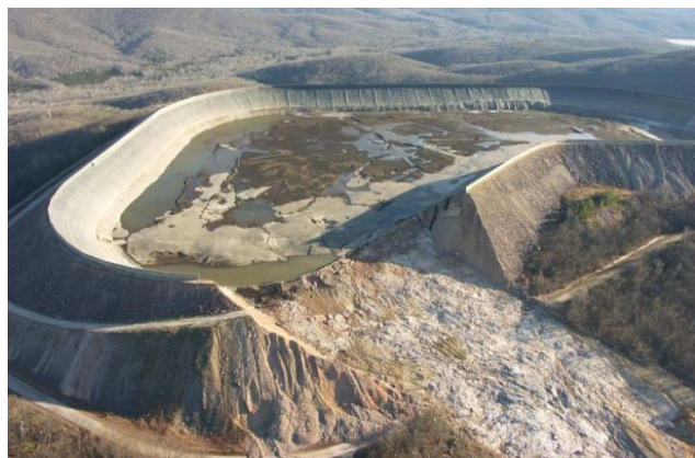
Photo 2.2 - Taum Sauk Upper Reservoir Dam
