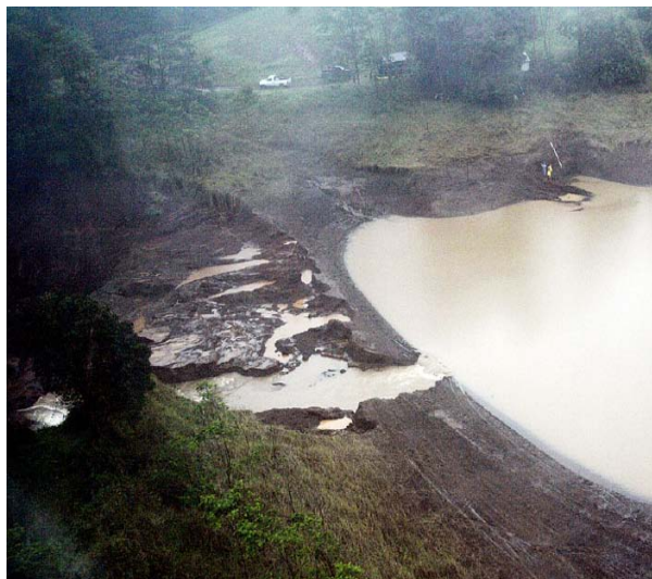
Photo 2.3 - Ka Loko Dam
