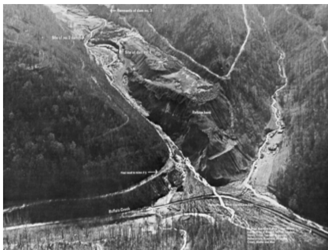
Photo 2.1 - Buffalo Creek Dam After Failure
