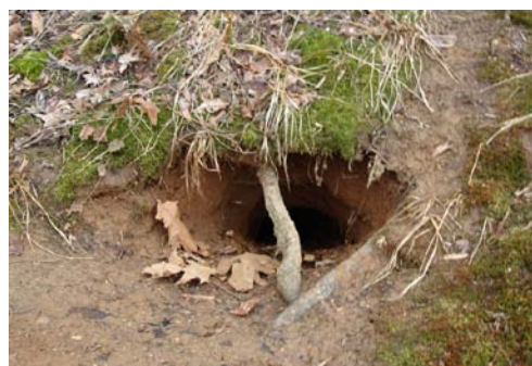
Figure 5-11 Embankment Animal Borrow (Rizzo Photo, 2007)
