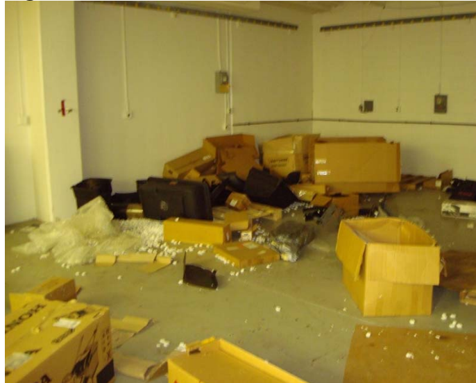
Figure 7: Room filled with debris
