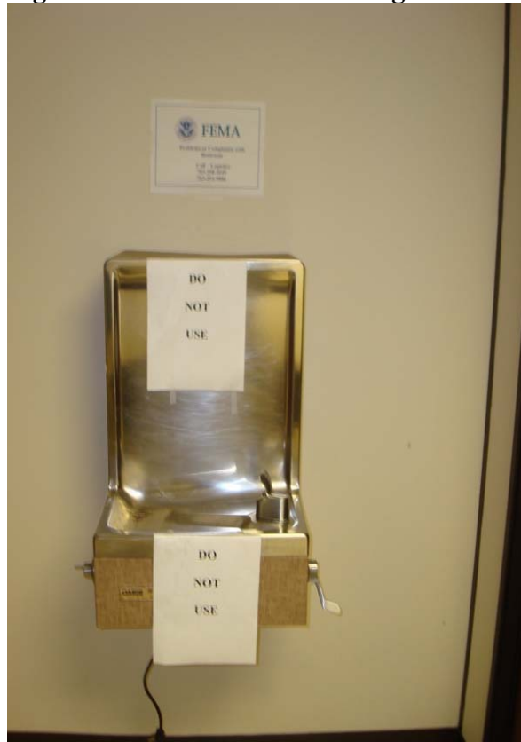
Figure 6: “Do not use” water sign on drinking fountain
