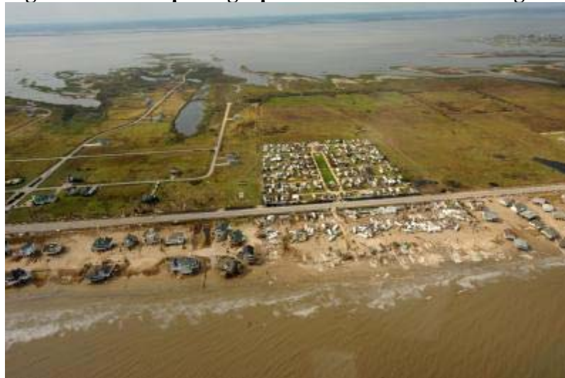
Figure 5: Aerial photograph of Hurricane Ike damage
