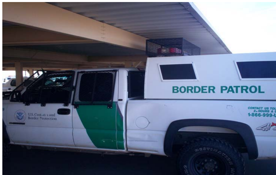
Figure 2. Examples of Carport Roofs Built Too Low for Border Patrol Vehicles
