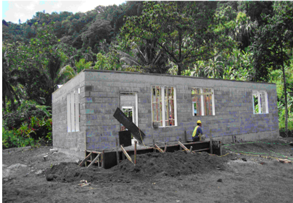
Figure 4. IA-TAC III permanent housing construction (American Samoa)
