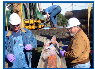
Contractor personnel evaluate core samples from a test boring at an ERT anomaly near Landfill 2.
