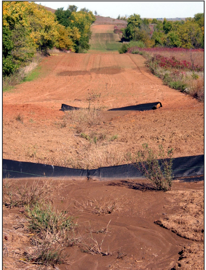
▲ Erosion control experiment on firebreak at the Kansas Training Center.
