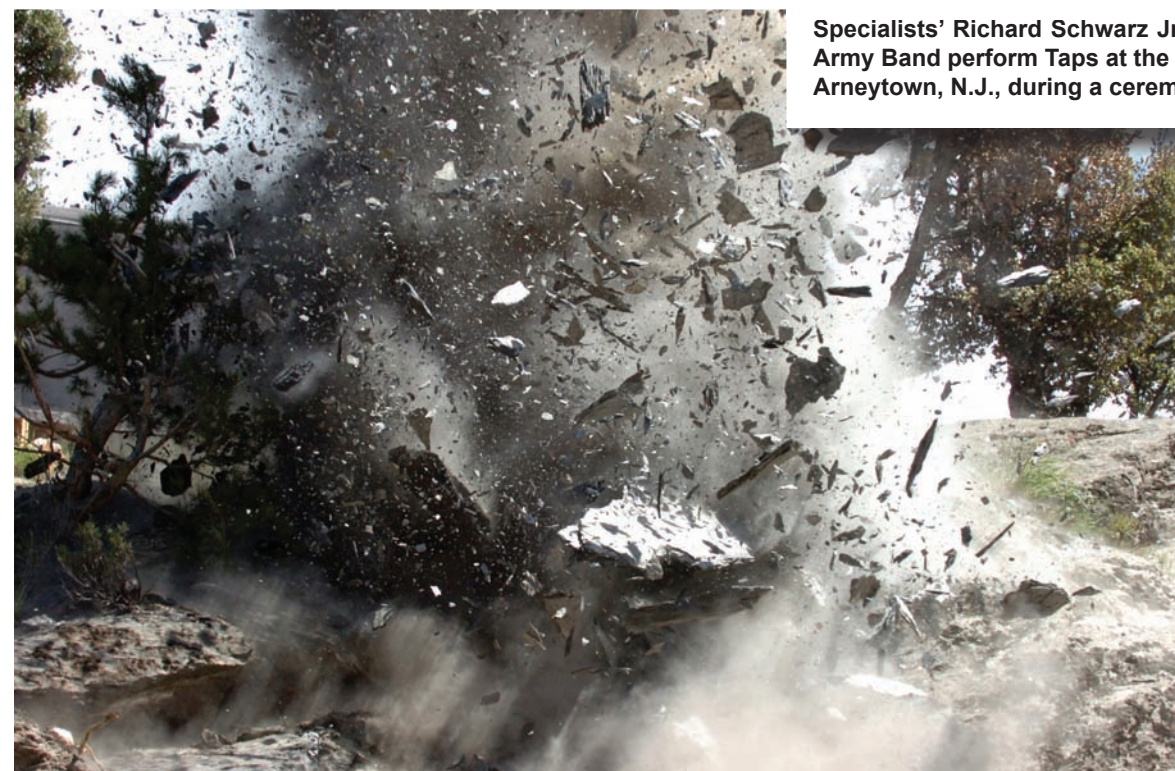
Combat engineers attached to B Company, 1st Battalion, 32nd Infantry Regiment, 10th Mountain Division, use controlled detonations to clear rock from a helicopter landing zone site at an outpost in the Nuristan province, Afghanistan. (Photo by Spc. Eric P. Jungels Jr.)
