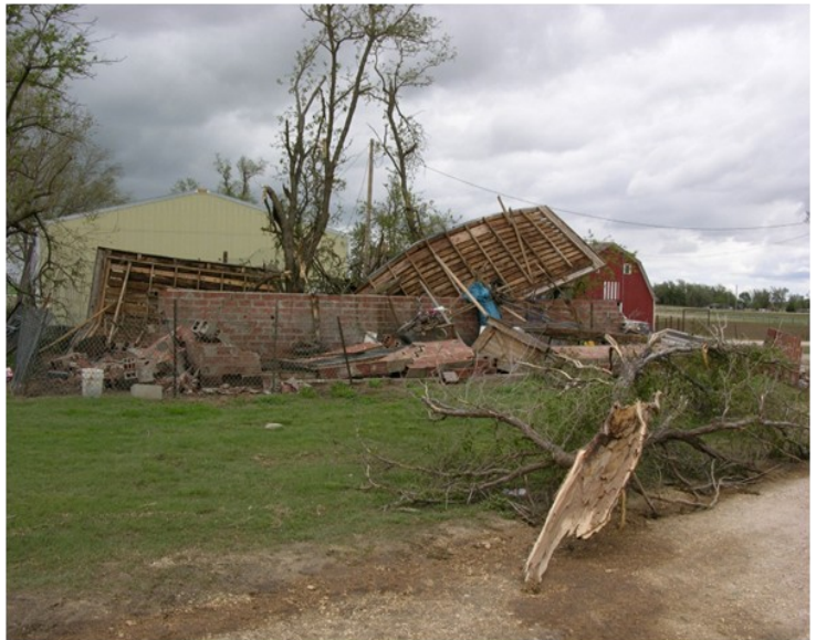
A destroyed shed and mangled tree was just some of the damage from an April 14 th tornado in the Tipton area. Photo courtesy of NWS Hastings.
