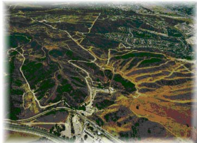
Aerial View of Landfill Remediation Site at Porta Bella, CA
