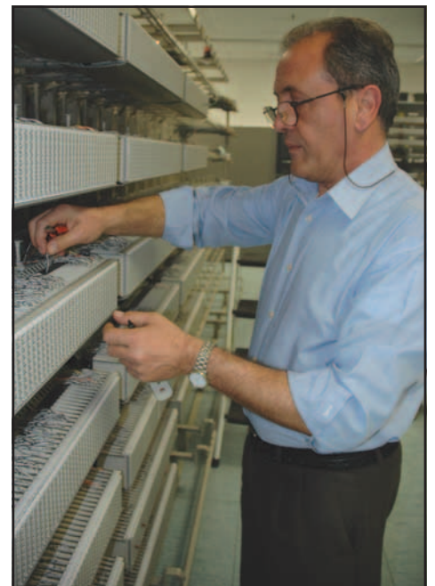
Raffaele Fusco, an Italian post employee who troubleshoots all problems in the switch room, works on installing a phone line in preparation for the new system. (Photo by Pfc. Crystal Abbott, SETAF Public Affairs)
