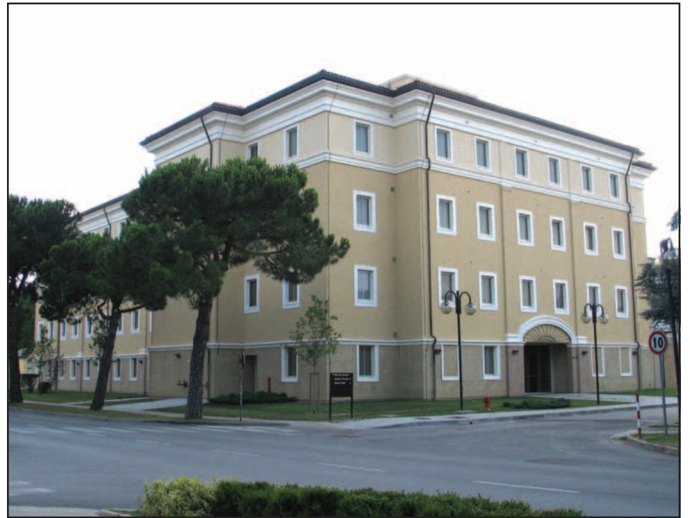
Above is one of two new LEED-certified barracks built for the 173d Airborne Brigade Combat Team Soldiers. (Photo by Diana Bahr, USAG Vicenza Public Affairs)
