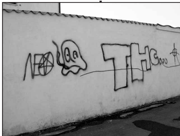
This is a picture of the graffiti damaging the last house on the left before leaving the Villaggio walk through gate.
