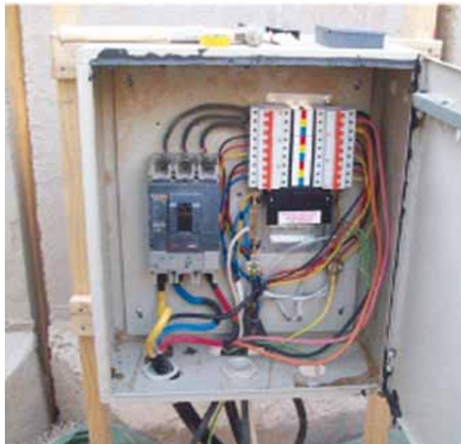
The before photo (L) depicts spliced and exposed wires serving as a makeshift distribution panel. The after photo (R) depicts the distribution panel after TF SAFE corrected the deficiencies according to NEC 2008 standards.
