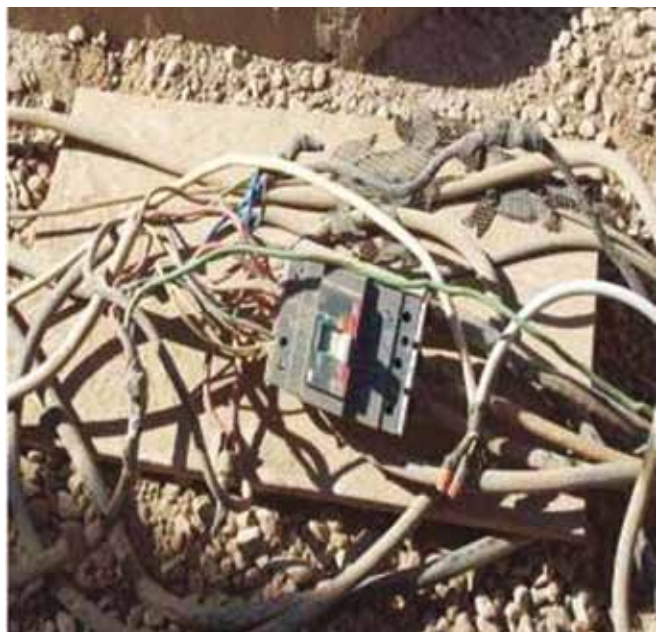
The before photo (L) depicts spliced and exposed wires serving as a makeshift distribution panel. The after photo (R) depicts the distribution panel after TF SAFE corrected the deficiencies according to NEC 2008 standards.
