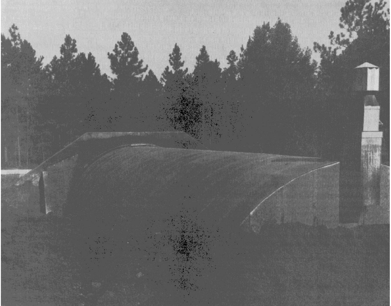
Figure 2-18. WATERPROOFING IGLOO—BACKFILL
