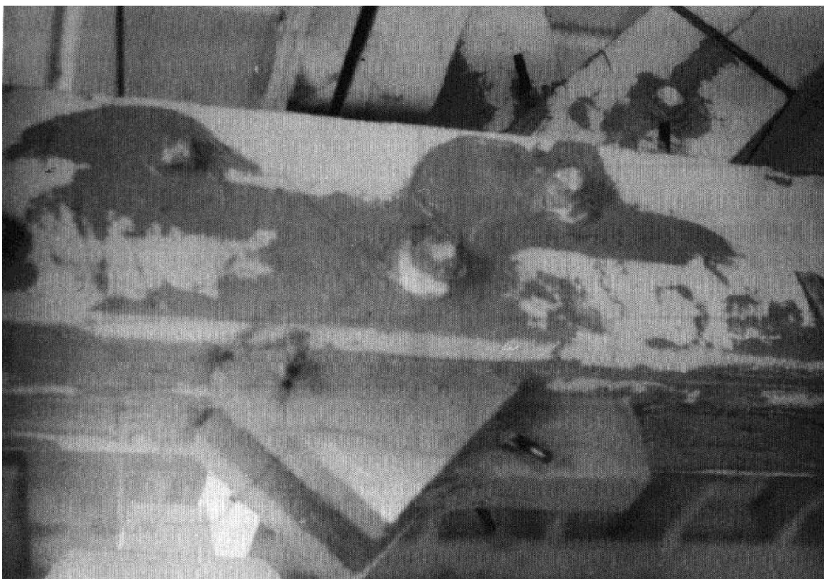
Figure 3-45. INSTALLED PORTS IN PLACE.
