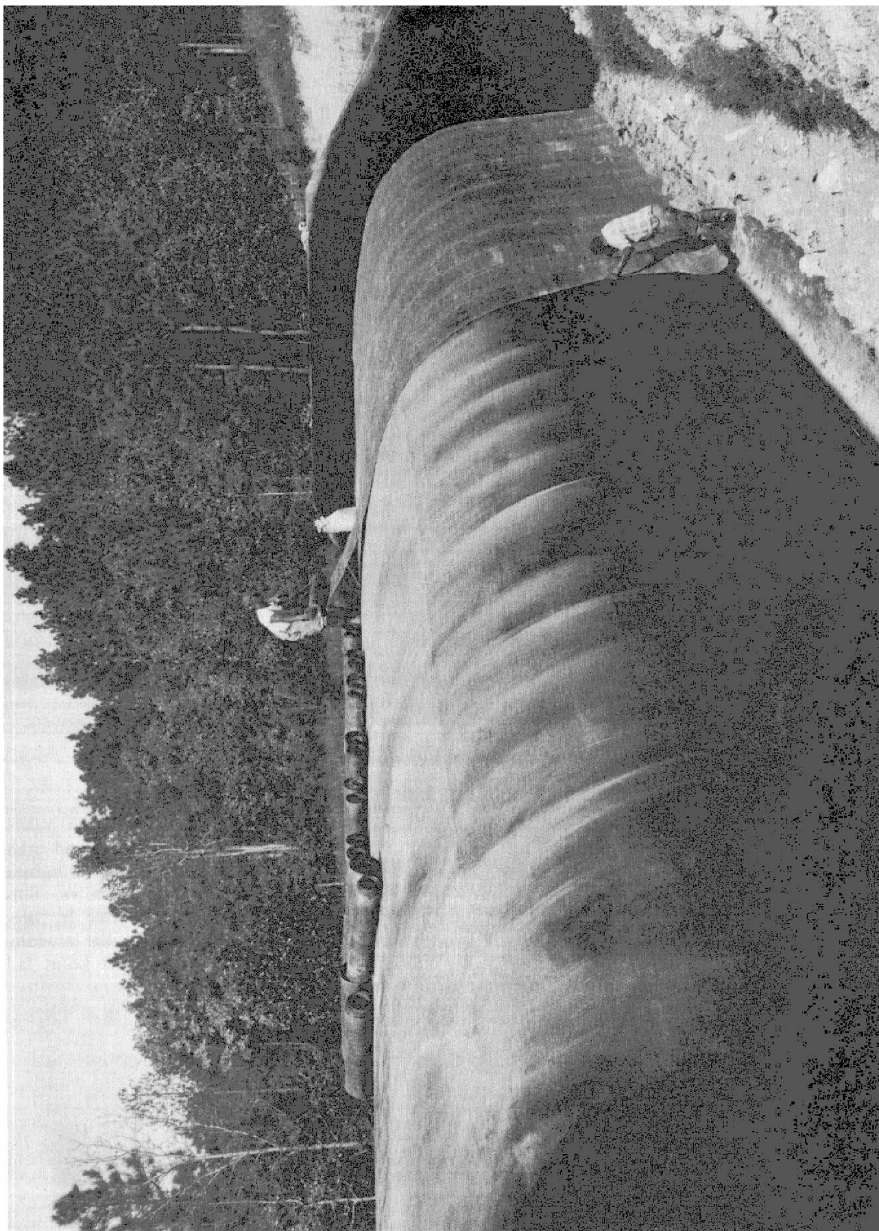
Figure 2-17. WATERPROOFING IGLOO—SLIP SHEET.
