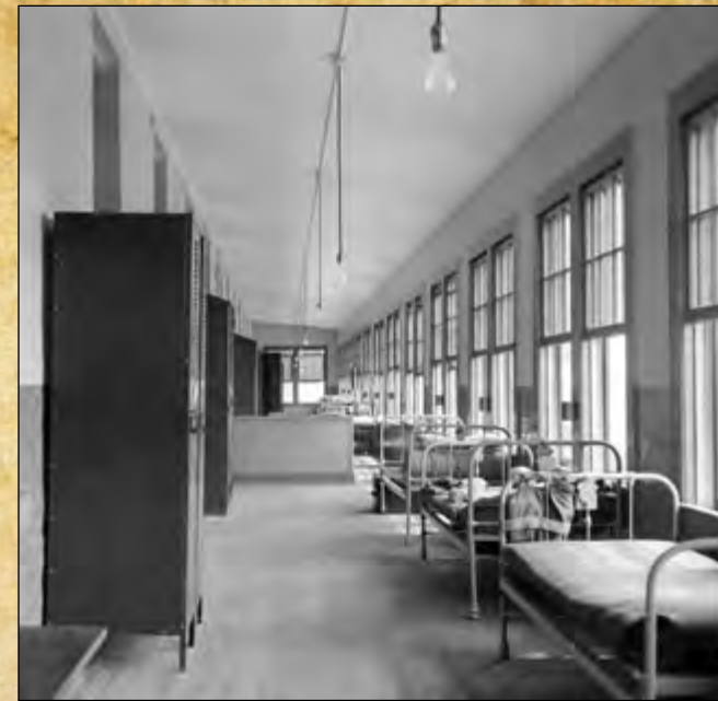
The Long Barracks porches were enclosed to provide additional billeting space, which eventually led to structural problems.
