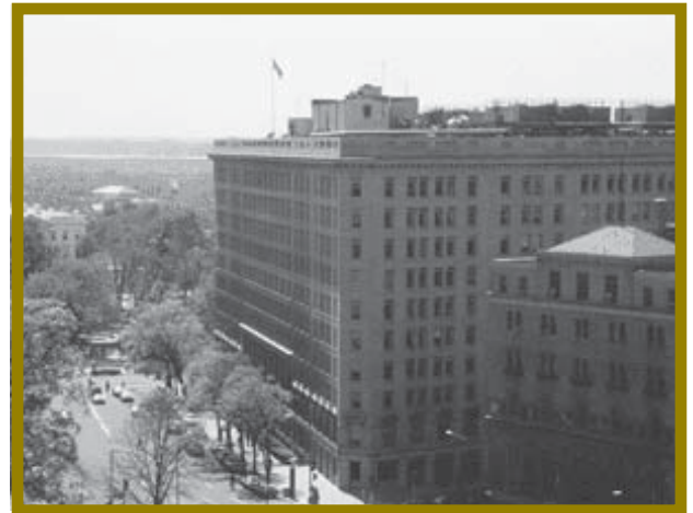
VA Central Office 810 Vermont Avenue, NW Washington, DC
