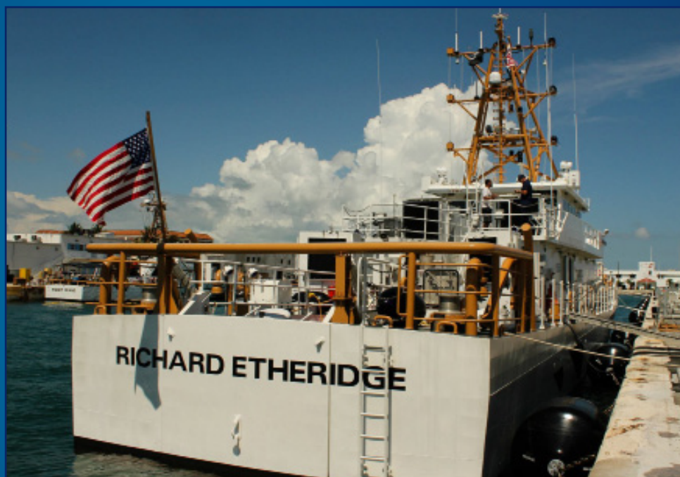
The Coast Guard Cutter Richard Etheridge is tied up at the refurbished pier at Sector Key West, Fla. The Major Acquisition Systems Infrastructure program ensured that critical waterfront infrastructure was in place to accommodate the six new 154-foot Fast Response Cutters that will be homeported there. U.S. Coast Guard photo by Petty Officer 2nd Class Michele Church.
