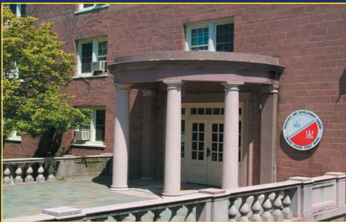
The USCG Research and Development Center's current home at the Avery Point campus of the University of Connecticut, Groton. (R&D Center Photo)
