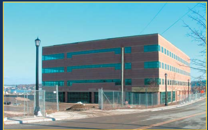
The Research and Development Center's new home, featuring 42,000 square feet of professional office space, is nearing completion at Fort Trumbull, New London, Conn. (R&D Center Photo)
