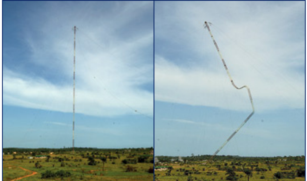
The Omega Navigation Tower in Liberia is observed before and during its controlled demolition. The 1,410-foot tall tower will go down in the Guinness Book of World Records as the tallest man-made structure felled by explosives. Photo courtesy of Gary Lehman with Tower Inspection Inc.
