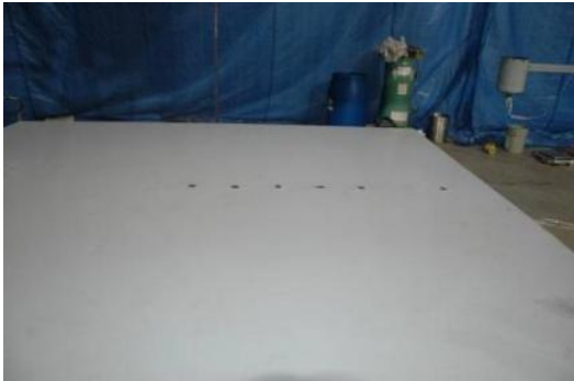
(c) – Coated Concrete
