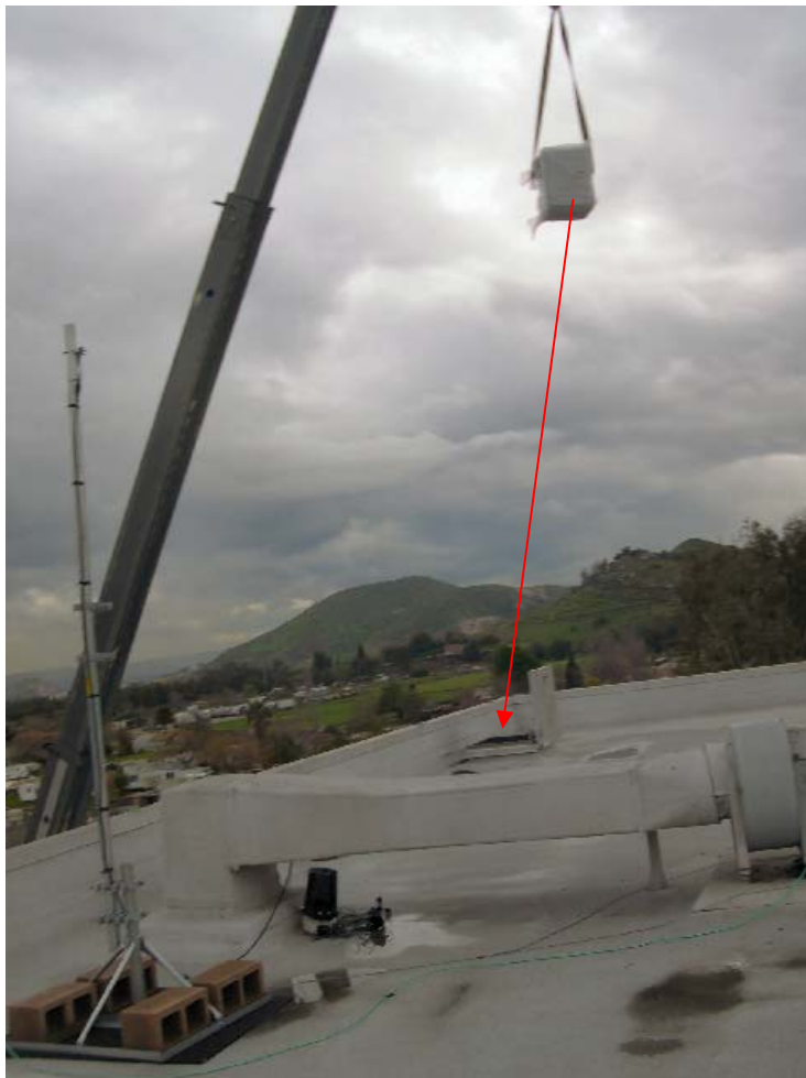
Figure 15: Roof Access for Receiver
